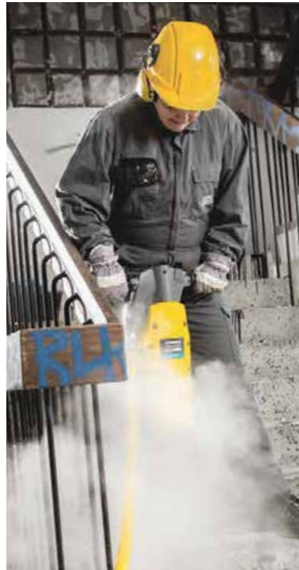
The Atlas Copco RTEX breakers feature reduced weight, vibration and air consumption vs. other breakers within the Atlas Copco product line. The RTEX35 weighs 73.2 pounds while the Atlas Copco P90S counterpart weighs 95 pounds.
